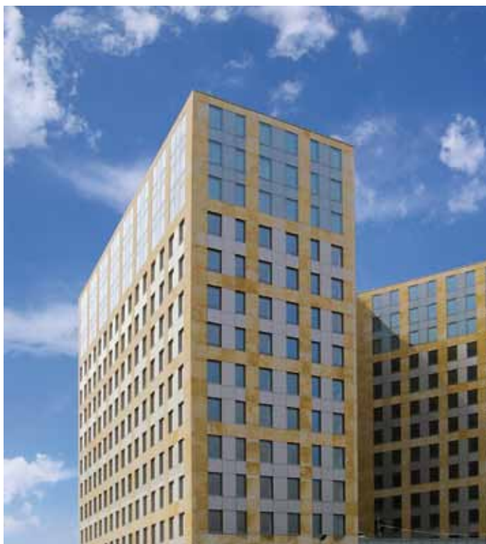
Office building IO – 1 Varsavia, Polonia
